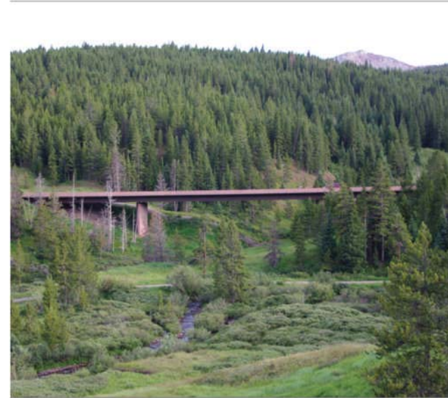
A | Roadway and bridge design should consider naturally occurring landforms and wildlife movement patterns.
