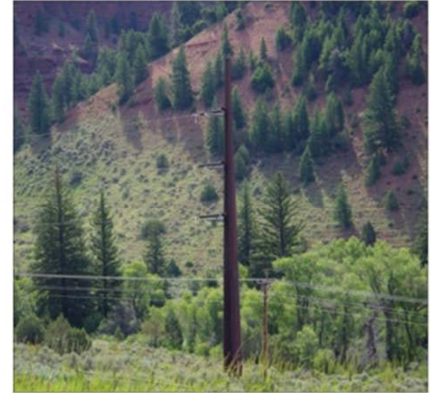
B | The application of color on these utility structures matches the surrounding landscape context.
