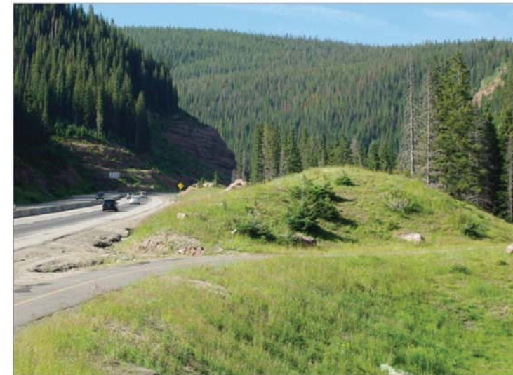
C | Utilize landform and planting within a buffer of at least 30 feet to protect recreational trails from the roadway.
