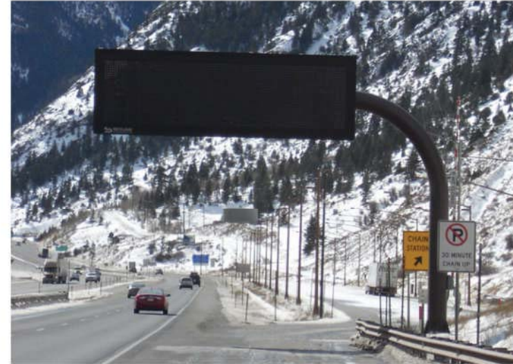
A | Single-arm monotube systems should be used.
