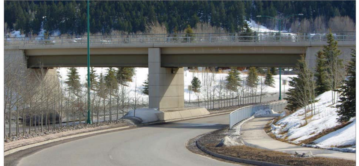
A | Safety and accessibility is improved by open, day-lit connections and a clear separation of vehicular and pedestrian circulation.
