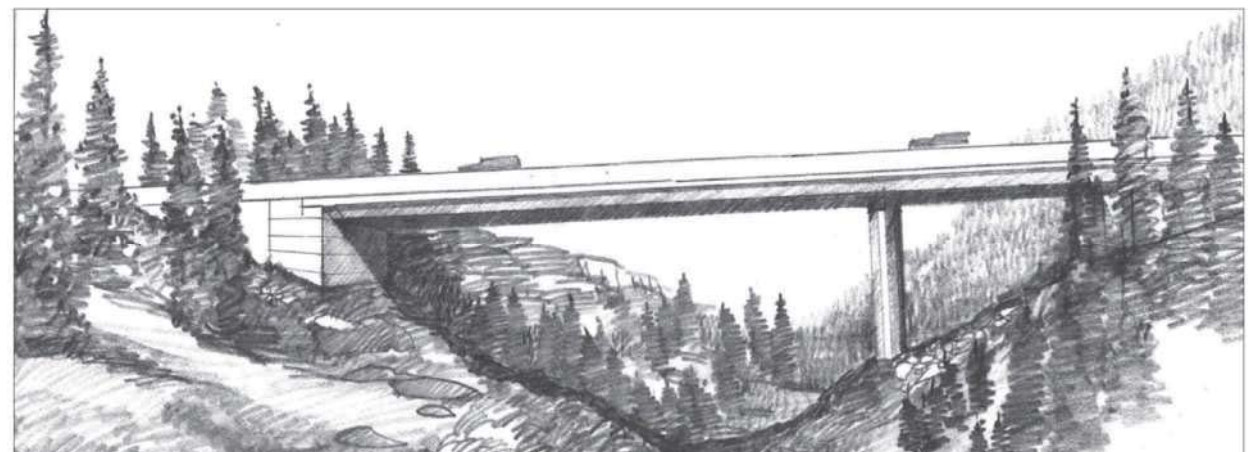
C | Open bridge solutions span significant landforms and stream corridors and leave undisturbed drainages below, minimizing environmental disturbance and impacts to the hydrologic and visual characteristics of the watershed.
