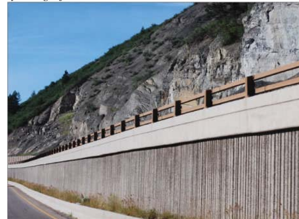
C | Where steep topography restricts median width, a vertical separation of at least 6' should be implemented.
