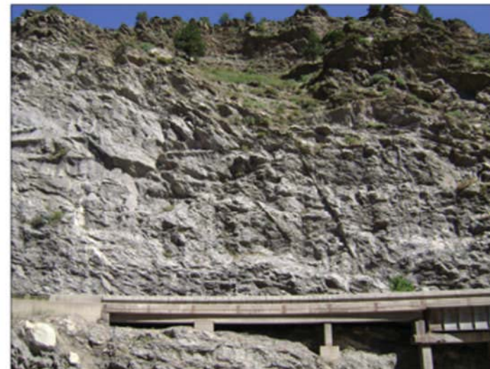
C | Disguise evidence of blasting technique along rock cut.
