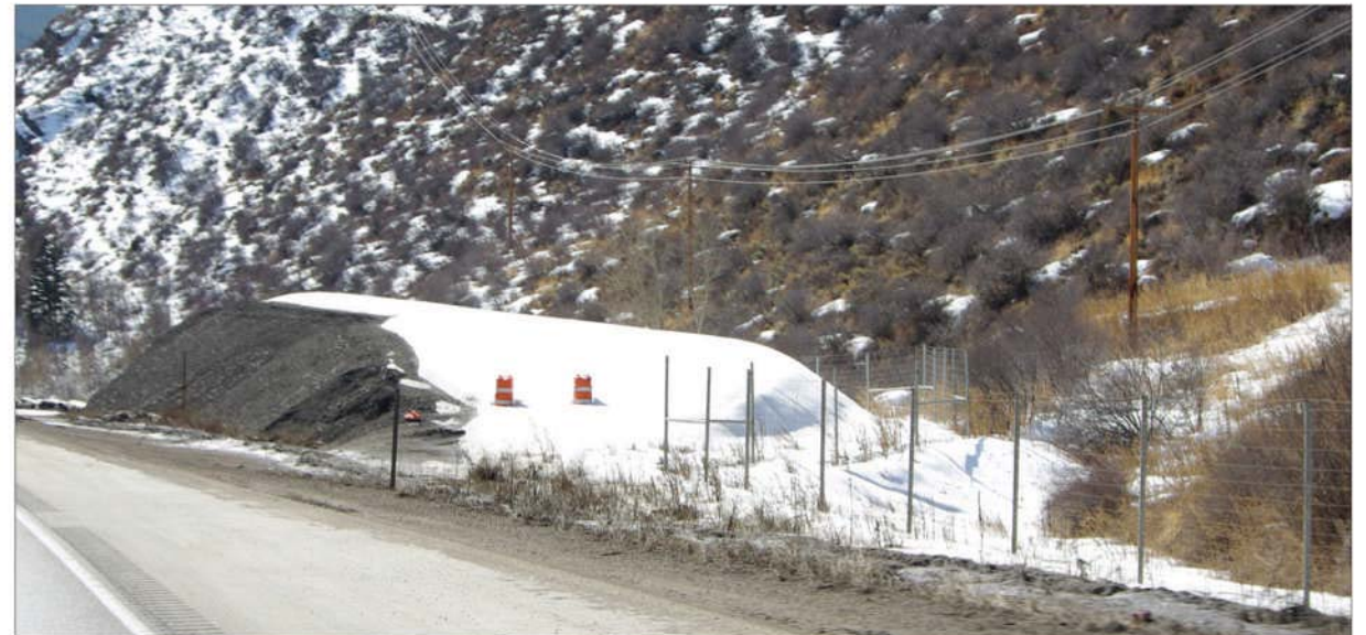
B | Construction and maintenance materials should not be stockpiled along medians or shoulders. This is especially important for areas with high visual or recreational value.
